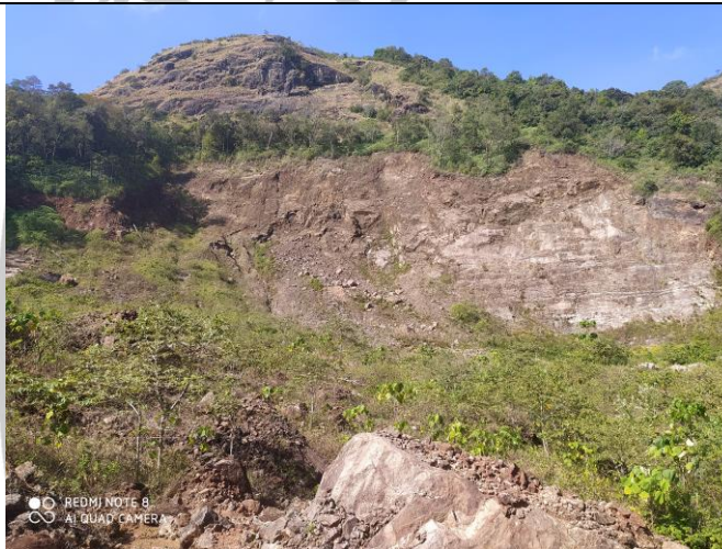
C) Rock cum debris flow in Thomara village (Tohra landslide) (12°09'52.06"N/75°43'32.71" E)
