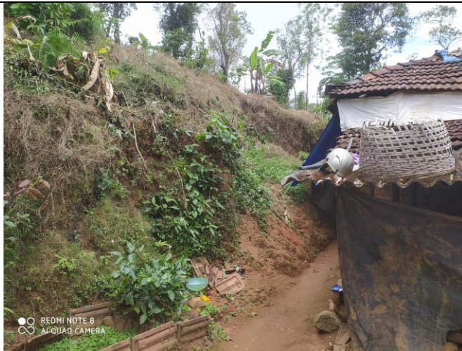
A) Cut-slope failure in Korthikad Thomara village (12°09'14.92"N/75°42'55.17"E)
