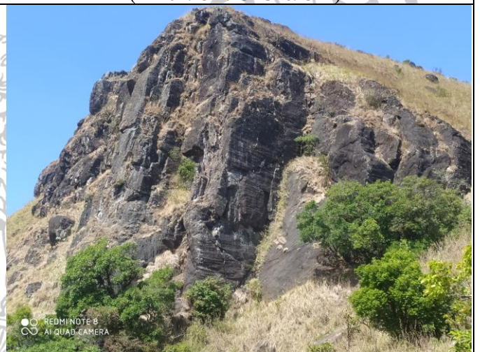
J) Rock wedge failure due to favorable joint interference (12°09'14.23"N/75°42'28.95"E)
