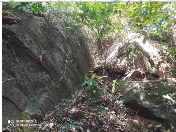
K) Rock wedge failure due to favorable joint interference (12°09'11.37"N/75°42'34.31"E)
