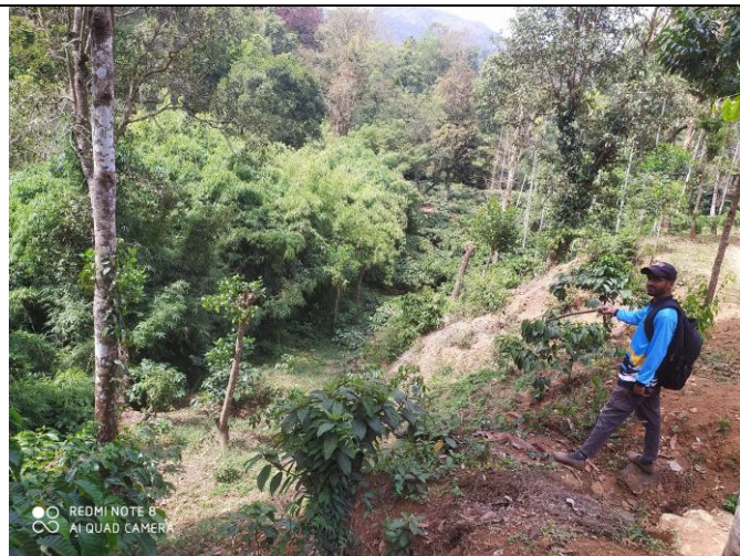
G) Debris slide occurred in Thomara village due to toe erosion (12°09'8.37"N/75°43'18.32"E)
